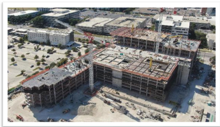
Uptown ATX - Block A Construction | 652,404 SF | Austin, TX
