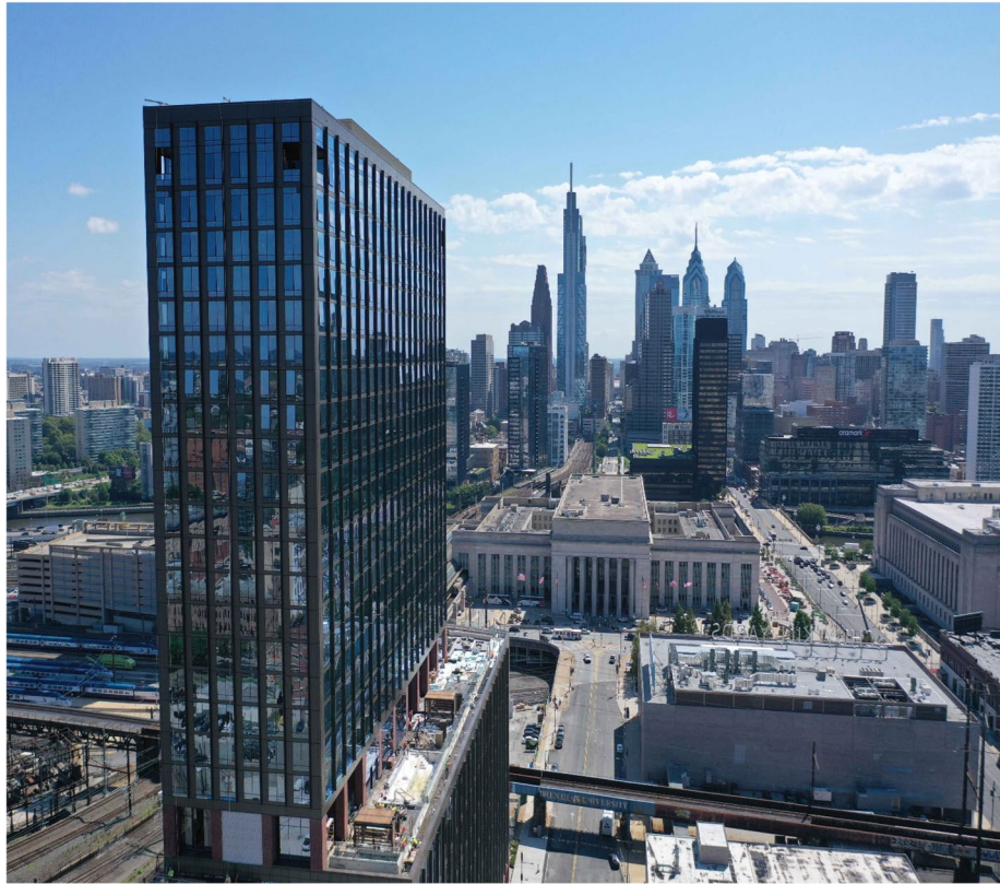
Above: 3025 JFK Blvd. Construction at Schuylkill Yards, Philadelphia, PA
