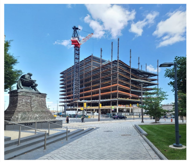
3151 Market Street (dedicated life science building), Schuylkill Yards, Philadelphia, PA
