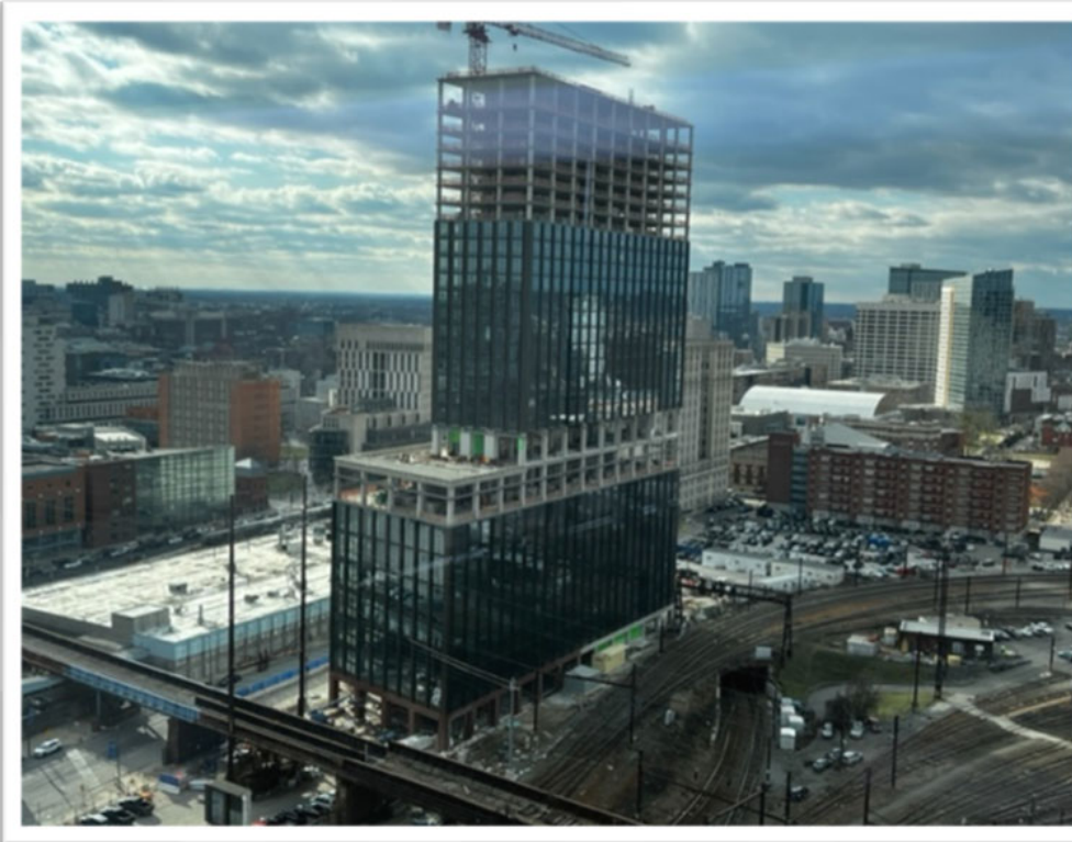
Above: 3025 JFK Construction | 570,000 SF | Philadelphia, PA
