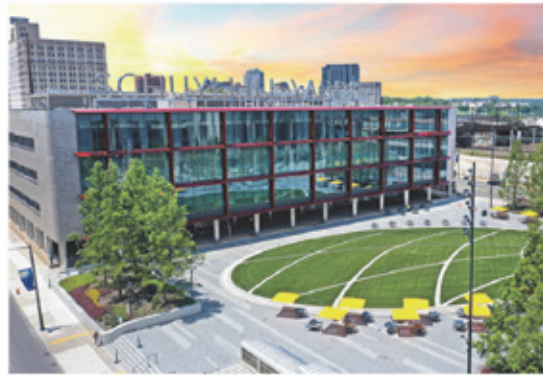
Redevelopment of Bulletin Building Philadelphia, PA
