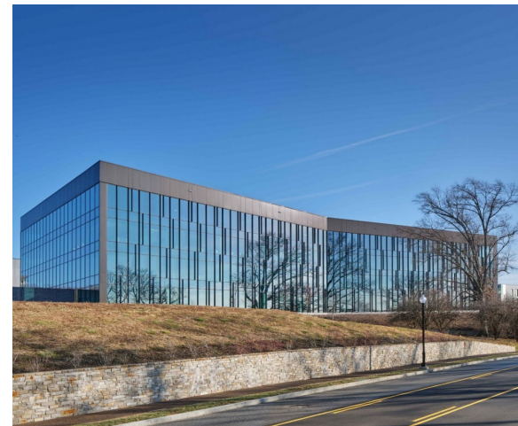
Arkema Inc. Headquarters - 155 King of Prussia Road, Radnor, PA
