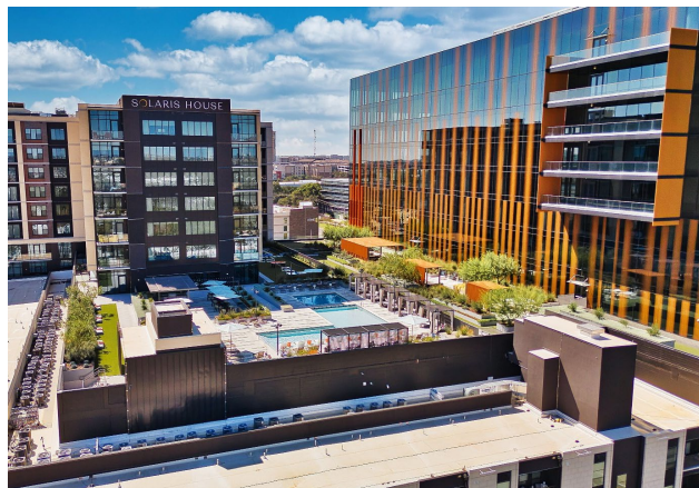
Uptown ATX - Solaris House | 652,404 SF | Austin, TX
